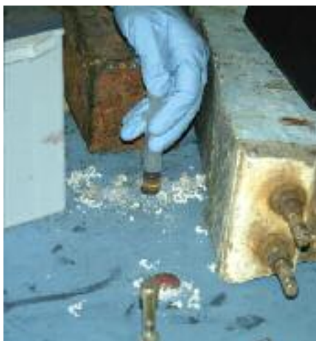
Filling a void with epoxy coming out of the exit hole
