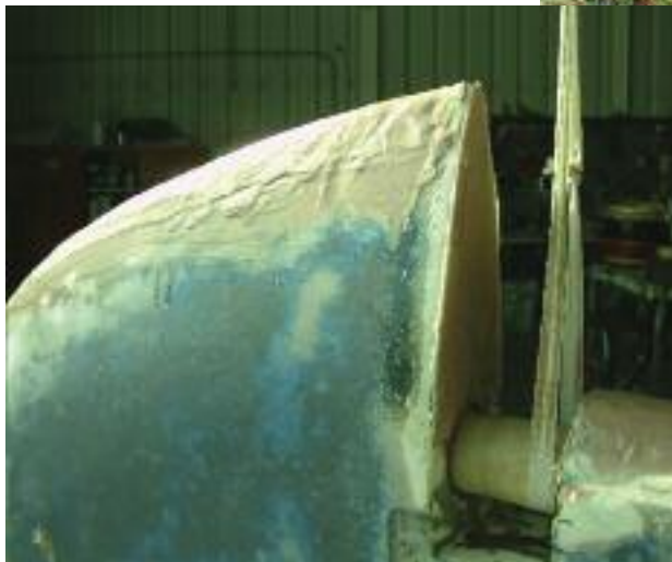
Edges taped and filled
