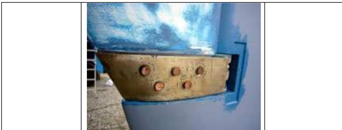
Once cut and numbered, the ends were annealed by heating to a dull red and quenched in water. This made forming the rivet heads an easier job. A 7lb hammer was held against one
